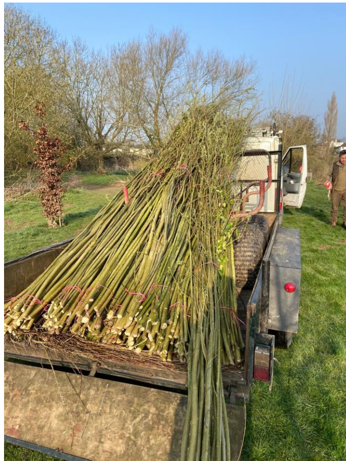
Erosion control – Willow Spiling
