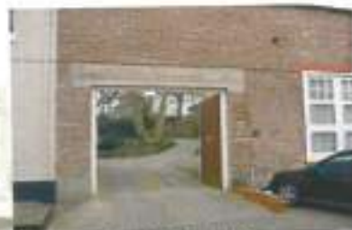
IMAGE 61 | EXPOSED ROUGH STONE
