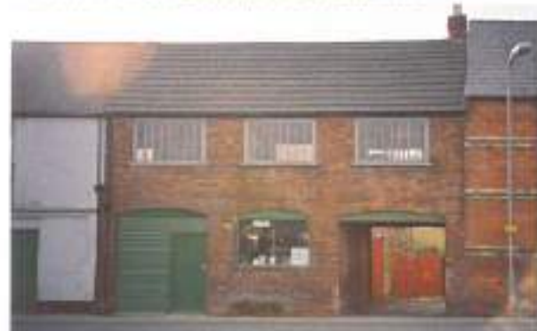
IMAGE 48: TWO STOREY TERRACED BUILDING - OVER GARAGE ENTRANCE
