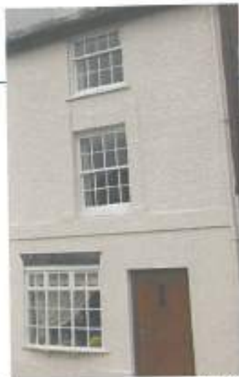
IMAGE 59 | PAINTED BRICK UPPER FLOOR, RENDERED GROUND FLOOR, DIMINISHING WINDOW SIZES
