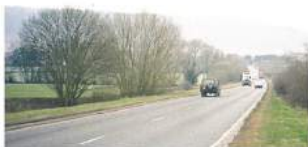
IMAGE 1: VIEW SOUTH ALONG THE A40 PAST THE SITE
