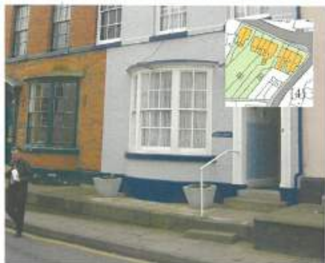
IMAGE 43 - THREE STOREY TERRACED BUILDINGS SET BACK BY 1M
