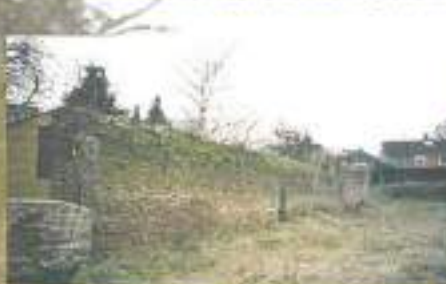
IMAGE 23 | FORD WALLS ON WESTERN BOUNDARY
